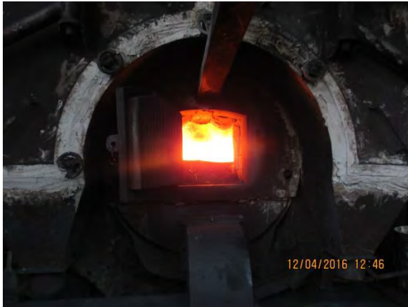
Caption: Boiler firing chamber at Simandhar Fabtex
